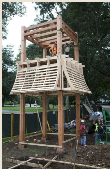
A belfry is under construction.
