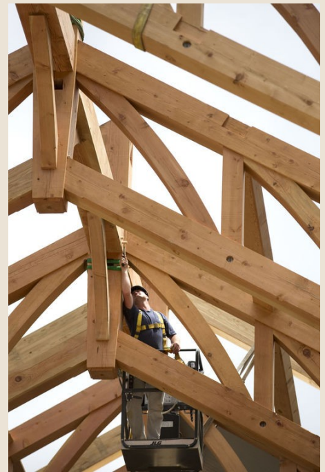
Ashley Cannon of Christiansburg-based Blue Ridge Timberwrights saws down the oak dowels for The Greenbrier's Chapel at The Greenbrier.
