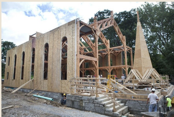
Blue Ridge Timberwrights based out of Christiansburg, Va., builds The Greenbrier's Chapel at The Greenbrier in White Sulphur Springs, W. Va. The timber frame structure consists of Douglas Fir wood.
