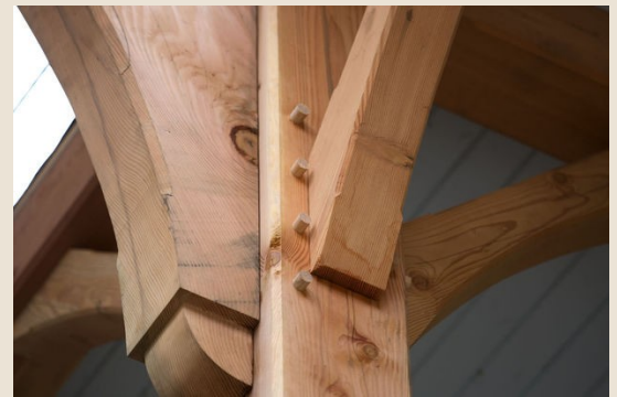
There are over 200 knee brace arches in the new chapel at The Greenbrier.
