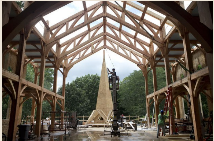
The chapel consists of nearly 800 pieces of Douglas fir.
