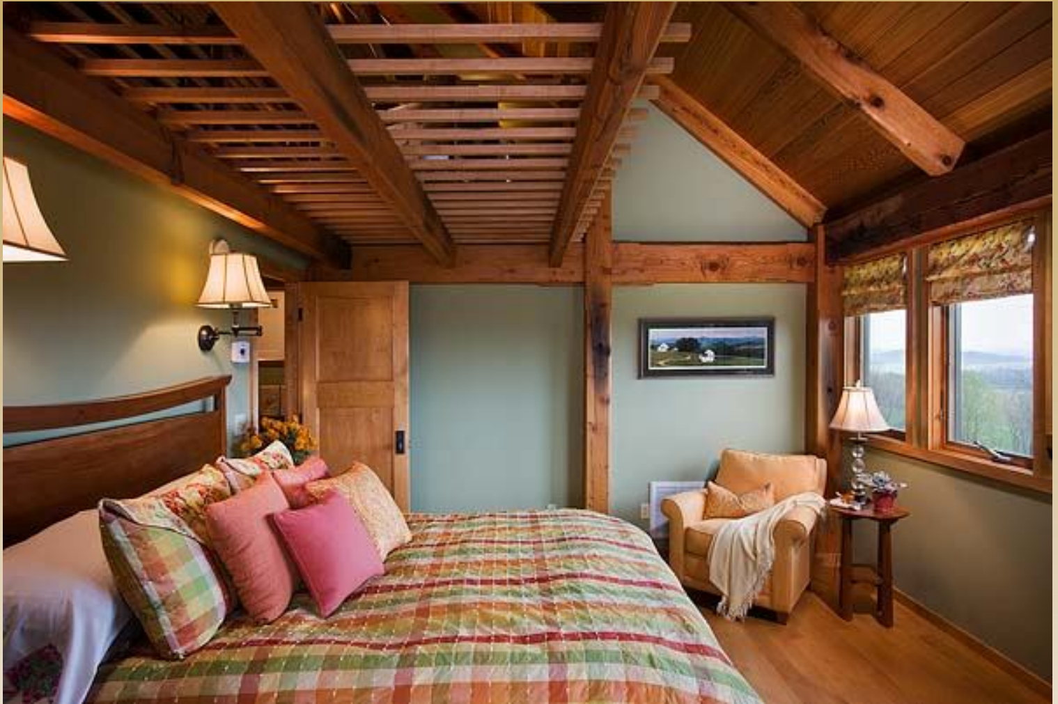
The loft bridge is constructed of Douglas fir in an open lattice pattern, contributing even further to the openness of the home by allowing Jim and Nancy a view of the timber frame loft ceiling from their master bedroom.
